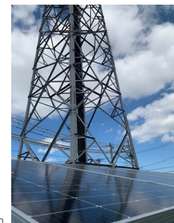
Sustainable Base Station
