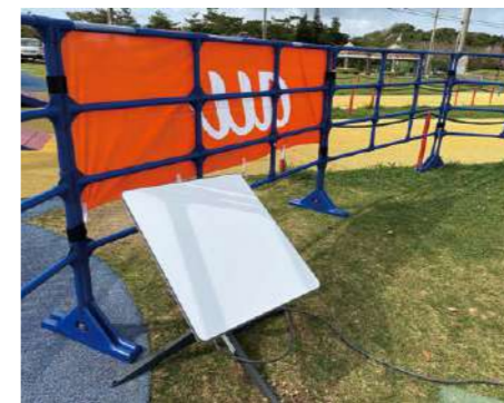
Installation of Starlink
